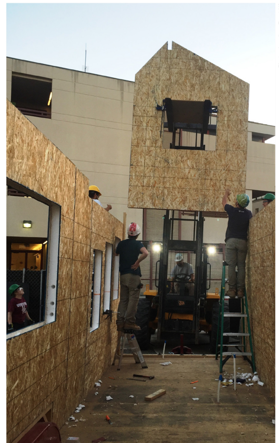
SCU's Tiny House takes shape as undergraduate teammates install the SIPs (Structural Insulated Panels).
